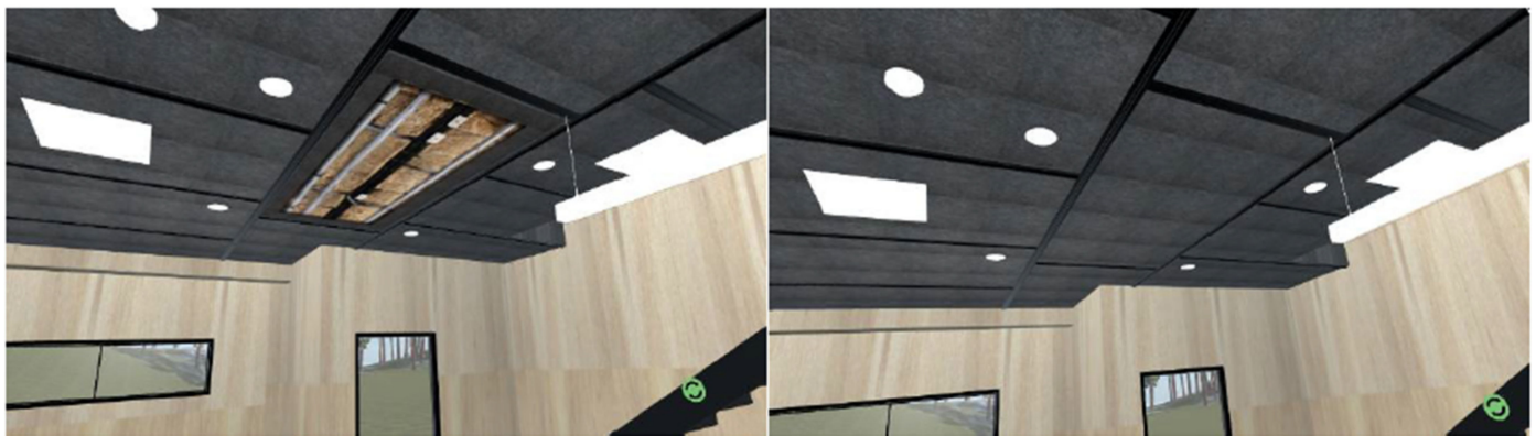
Figure 10. Acoustic felt ceiling panels reveal insulation and allow access to mechanical and electrical plant services throughout the multiple lifecycles of the building.
