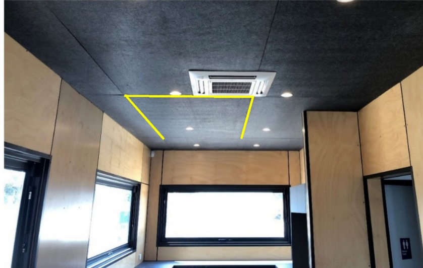
Figure 3. Disassemblable and resilient ceiling and cladding.
