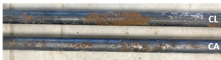
Figure 5.16: Visual inspection of rebar
