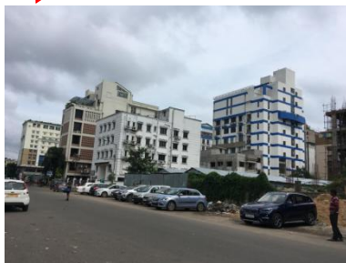
Image 5 showing very few commuters on the road in the evening
