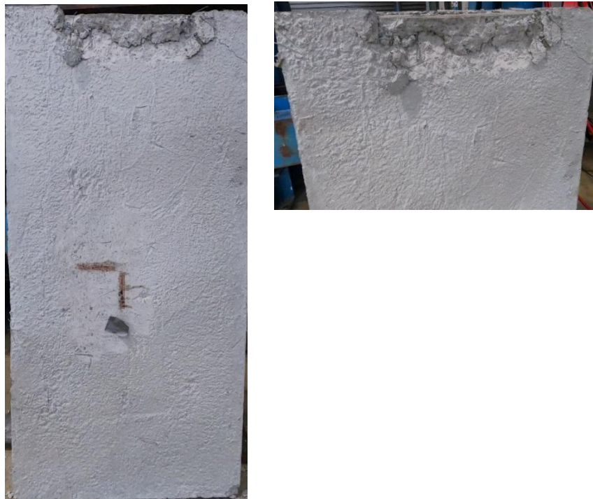
Figure 7-17 Concrete damage under compression at ultimate failure
