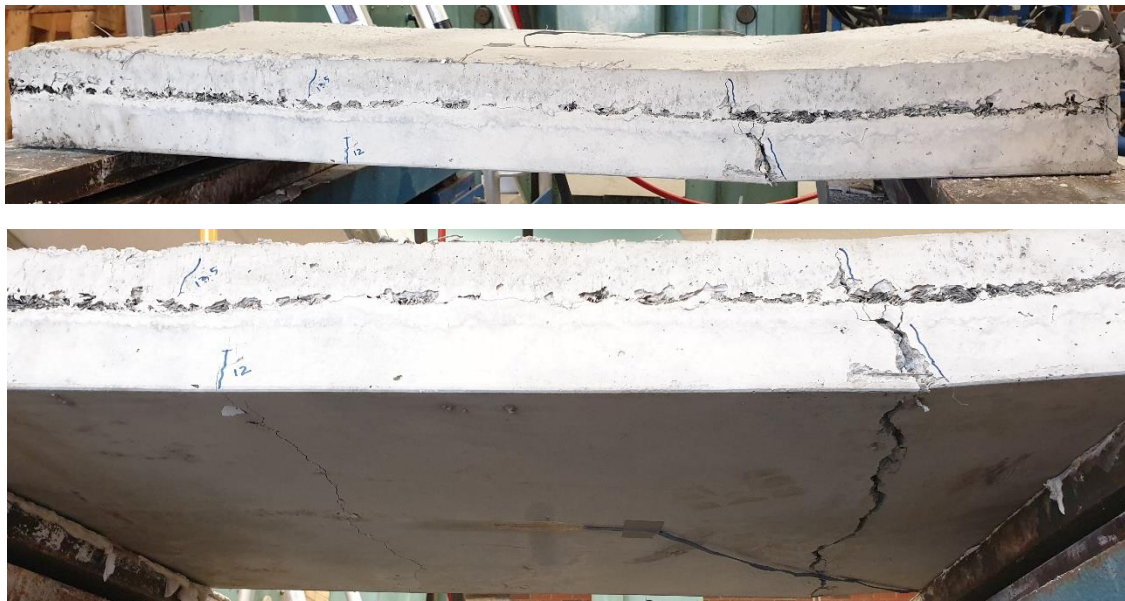
Figure 7-12 Concrete damage - flexural failure in the panel
