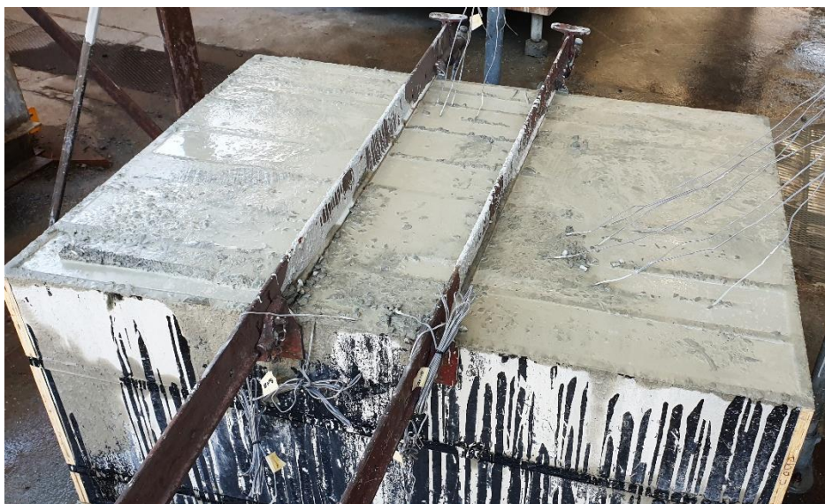
Figure 5-5 Formwork and casting of all concrete panels
