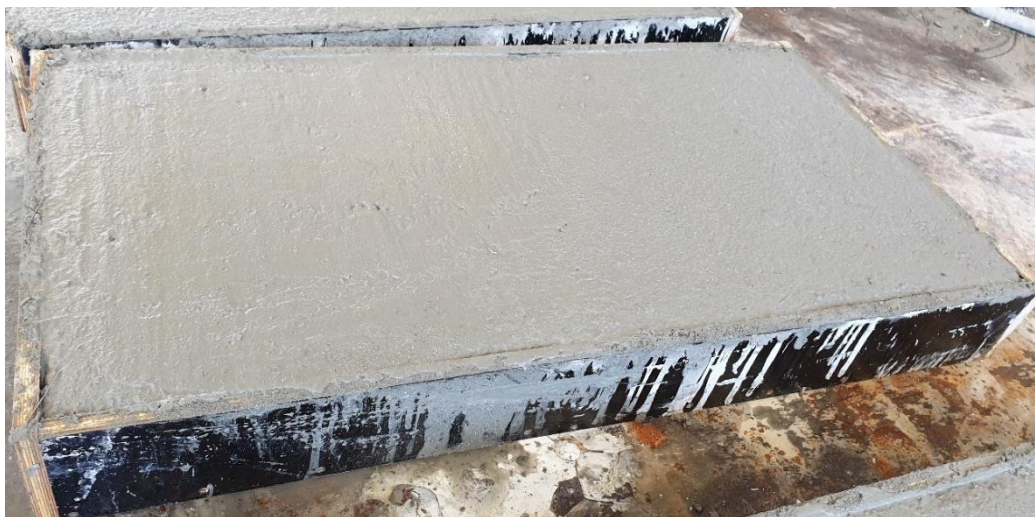
Figure 7-4 Formwork and casting of panels
