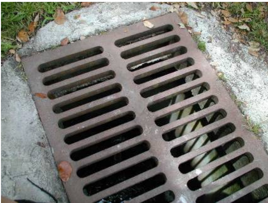
Drains were filled with debris and frogs, too.
