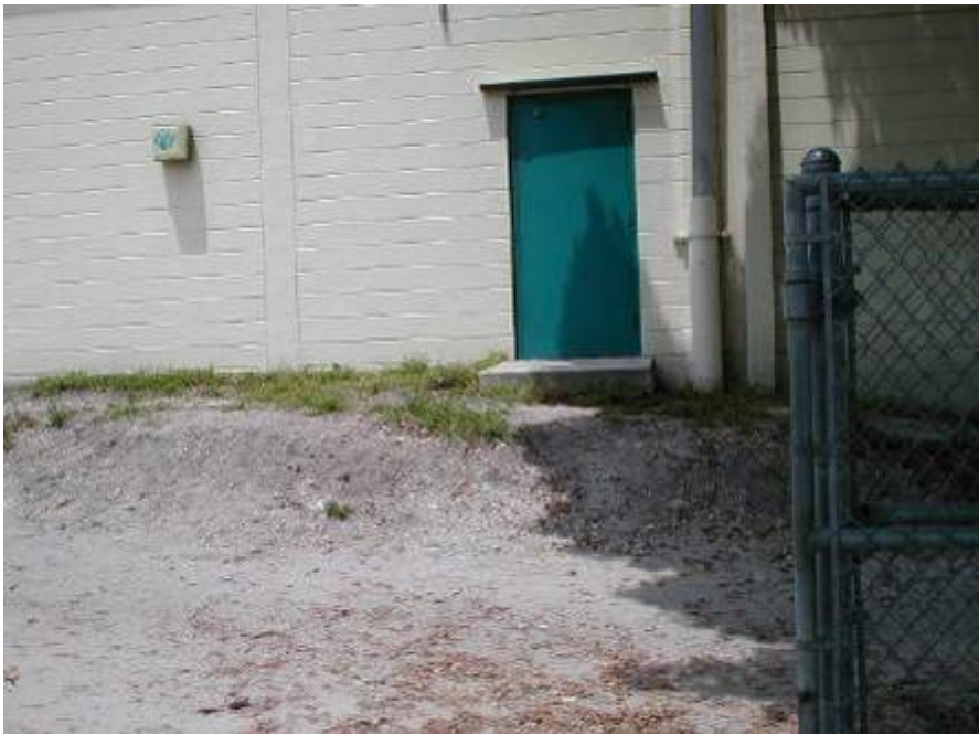
Ground was eroding under classroom building.
