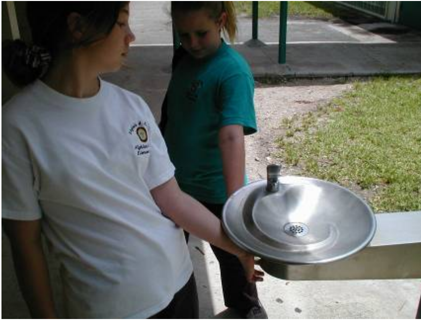
Water fountain dripped and wasted water.
