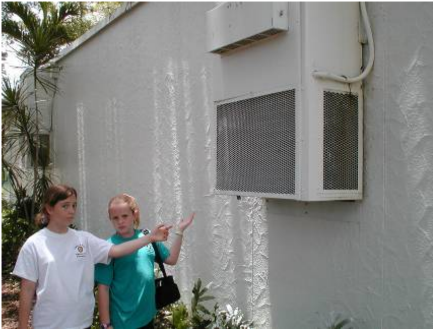
Air conditioner puts out very hot air outside of the building.
