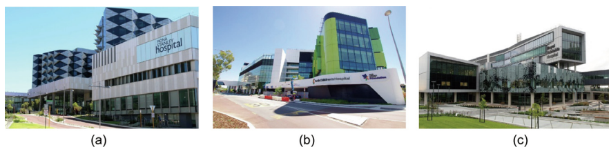
Fig. 2. Three Australian hospital mega-projects. (a) FSH; (b) PCH; (c) nRAH.
