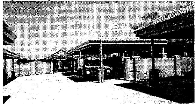
Carports shade northerly glazing to Dwellings 4C and 4H
