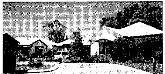
Dwellings 7B and 7C have northerly orientation but eaves and plants block a significant amount of direct solar radiation
