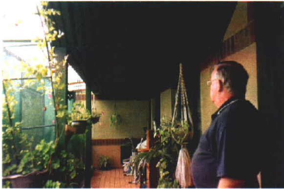
Figure 5-1 An extended canopy on all dwellings blocks both summer and winter sun from northerly windows (Development 1)
