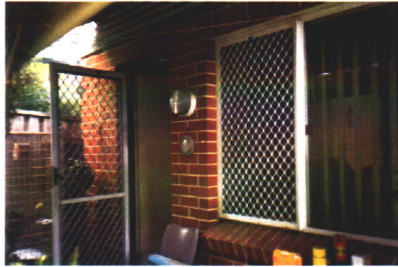
Figure 7-1 Typical security grills in front of doors and operable windows
