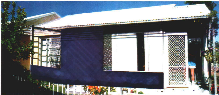
Figure 8-1 Possible changes to appearance of existing dwelling (upper image) with a Trombe-Michel wall incorporated (lower image)
