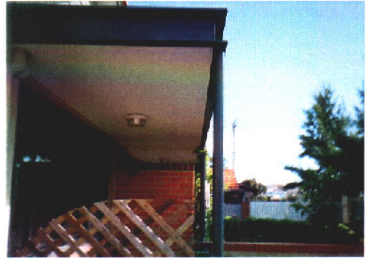
Figure 5-2 Extended eaves block significant winter sun from glazing (Development 2)
