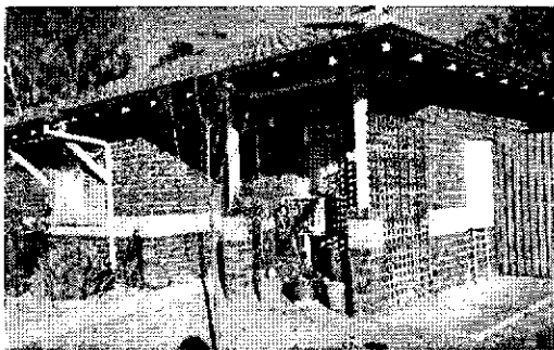
Dwelling 3A – significant shading of northerly glazing to living area in winter
