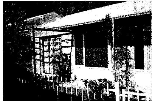
Dwelling 5D – no shading to northerly bed room window and significant shading to living room window
