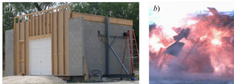
Fig. 7 Hydrogen deflagrations in a garage: a) before the explosion; b) during the test [71]
