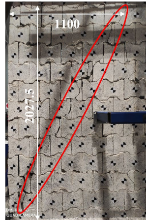
c) Diagonal crack on the left of the wall at 50mm lateral displacement
