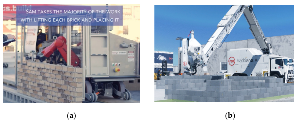
Figure 9. Brick laying robotic systems. (a) SAM 100 [140]. (b) Hadrian X [141].
