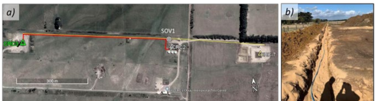
Figure 1 (a) Location of the buried HWC cable (yellow) and CO 2 pipeline (red) at Otway site. (b) A photo of HWC in the trench, the pipeline is buried 0.4 m below the cable.
