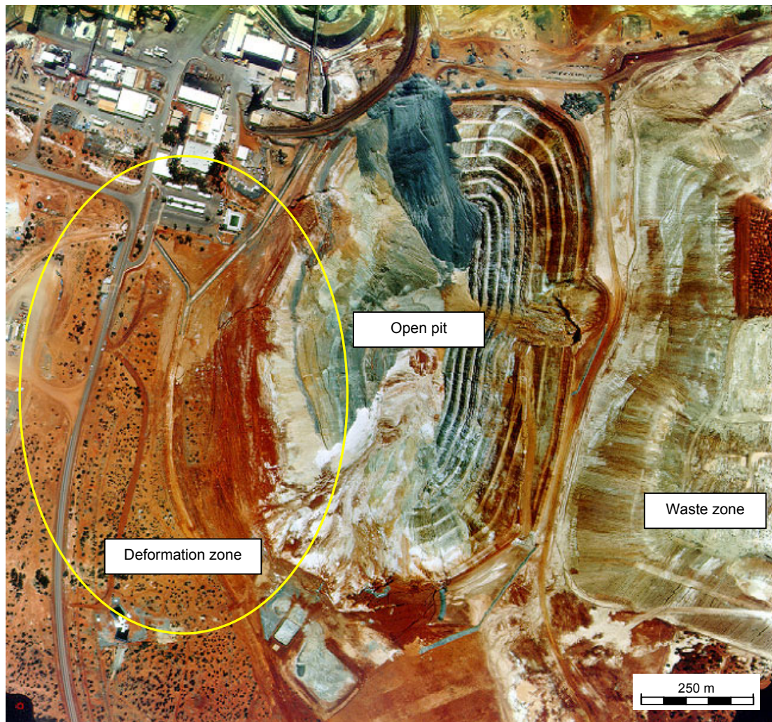
Figure 3.3 Aerial photograph showing the Leinster mine site taken in 2001. Sparse vegetation cover over the deformation zone can be seen.
