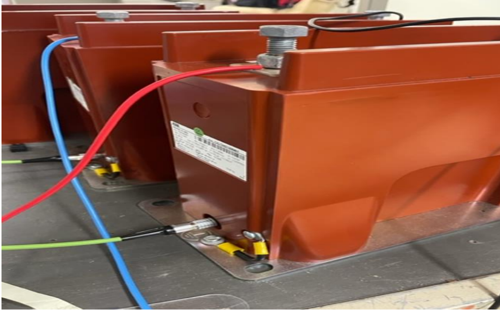
Fig. 5.9. NCIT – ABB make KEVCD combi-sensor.
