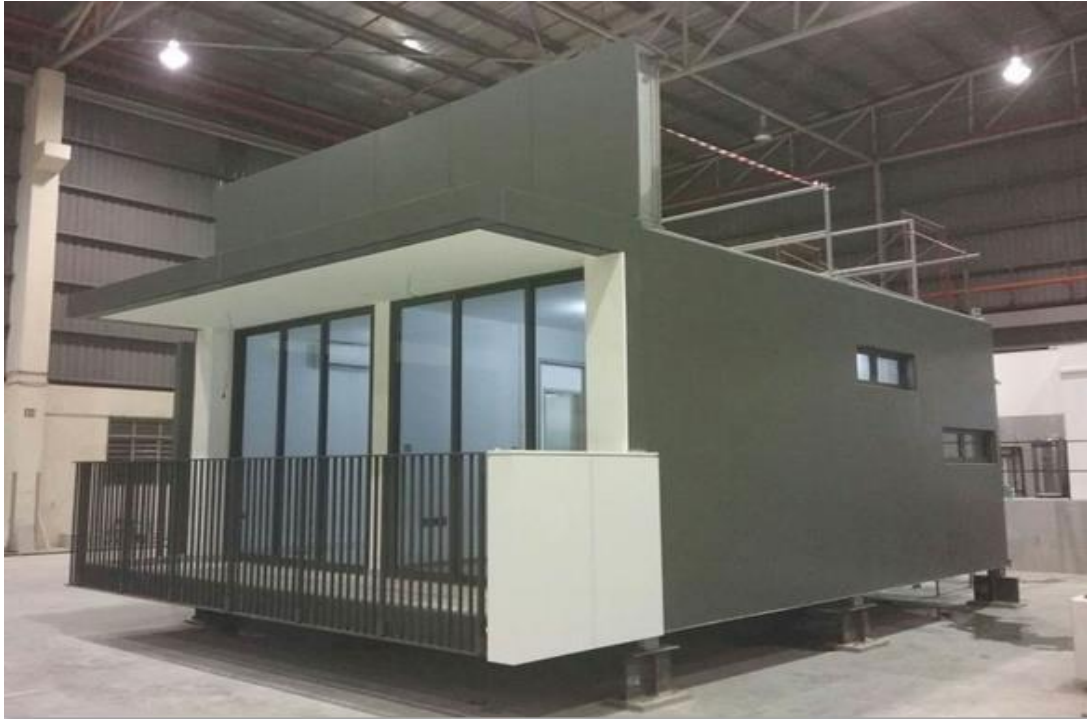
Figure 5.26 Completed module at the warehouse
