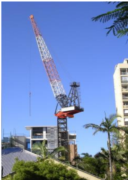
Figure 5.13 Luffing tower crane (L), and hammerhead tower crane © (Workplace Health and Safety Queensland, 2017)
