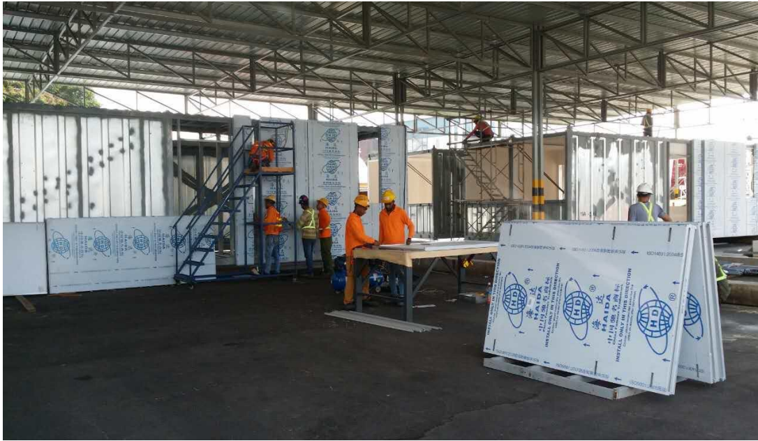
Figure 5.3 Module production at an off-site factory
