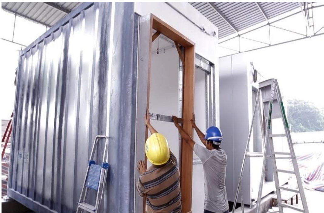
Figure 5.21 Door installation
