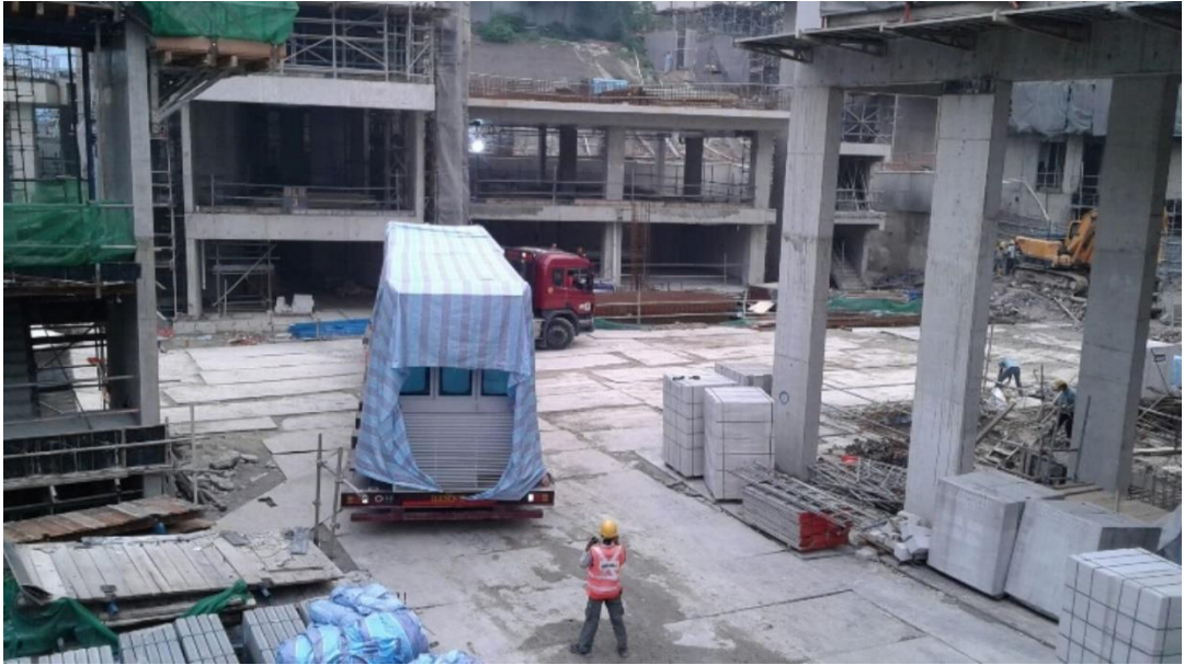
Figure 5.31 PPVC module at the construction site
