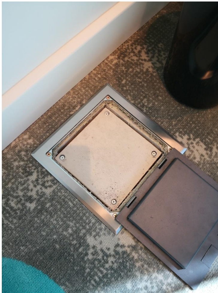
Figure 5.36 Installation and inspection hole for inter-module connection
