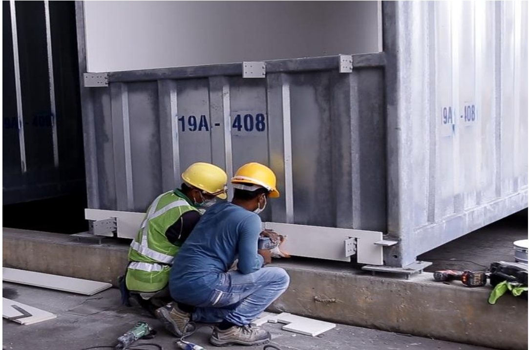
Figure 5.20 Fireboard installation
