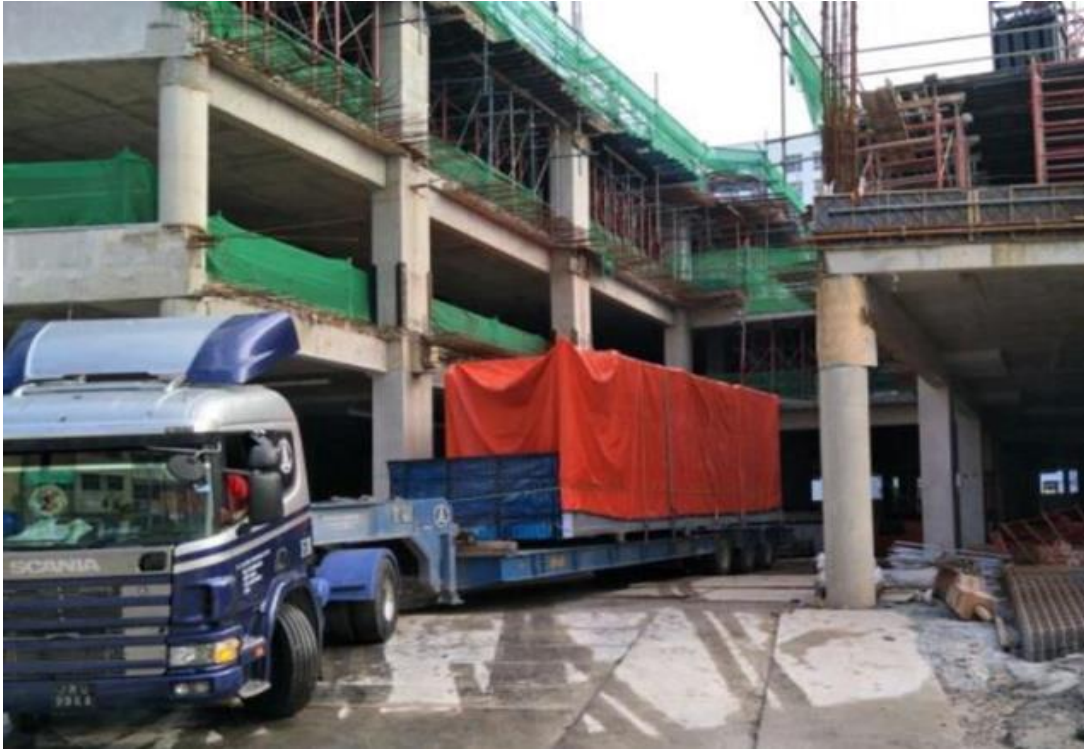
Figure 5.14 Arrival of the PPVC module at the launch area
