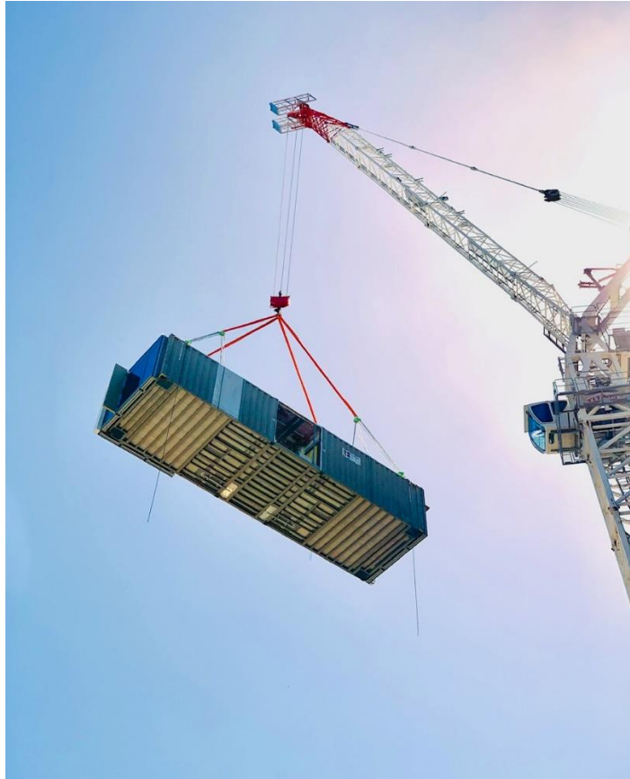
Figure 5.34 Luffing tower crane in project 2
