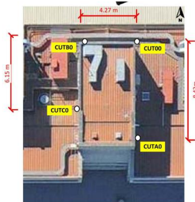
Plane view of CORS on top of building 402 – Curtin University
