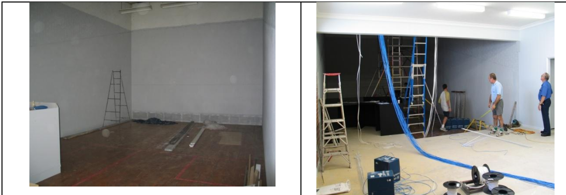
Figure 5a. Renovation of the NMRS Squash Court
