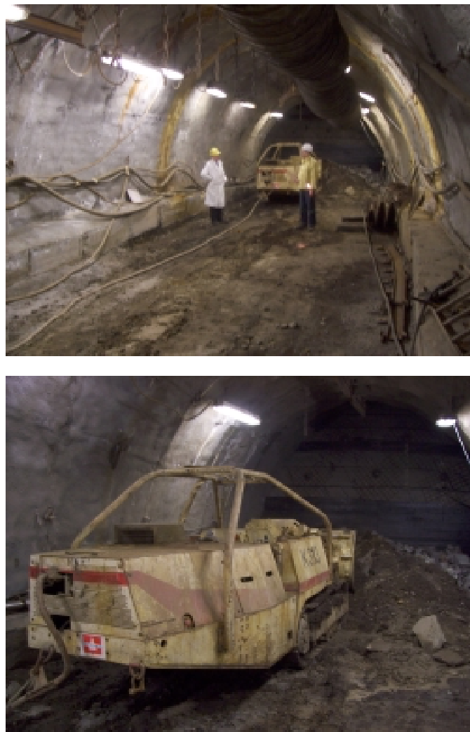
Figure 12. The underground training mine for a drill and blast operation at DSK.
