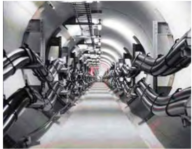
Figure 23. Cable Tunnel Installation (Nexans / CIGRE 2017 [12])
