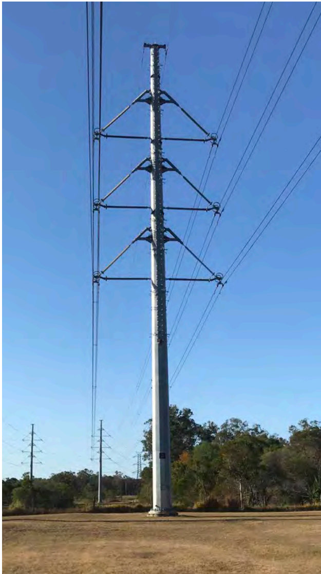
Figure 6. 275kV Double Circuit Compact Steel Pole
