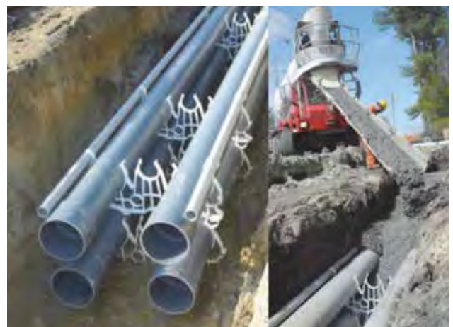
Figure 27 2x2 duct bank (left) and concrete backfill installation (right) [31]
