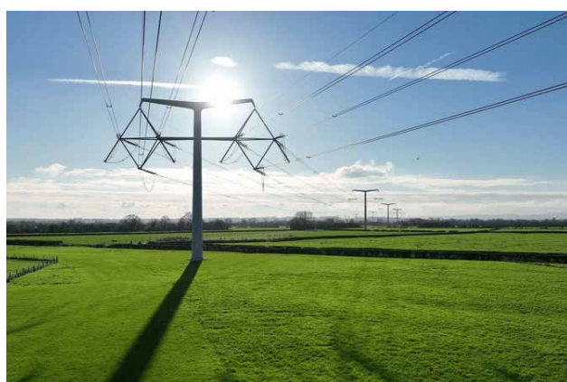
Figure 26. Hinkley Point C Project - 400kV T-Pylon structures (National Grid)
