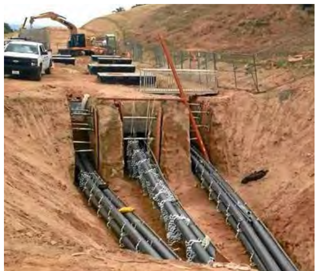
Figure 7. Tehachapi 500kV Underground Cable Installation (dailybulletin.com)
