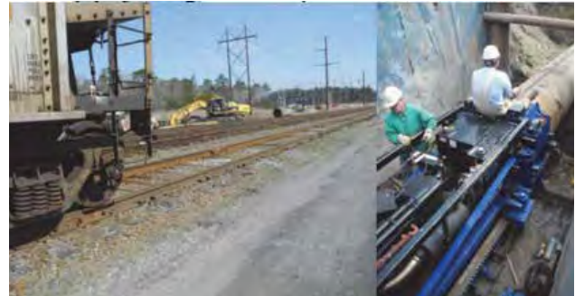
Figure 29 Pipe-jacking operation under rail sidings [31]
