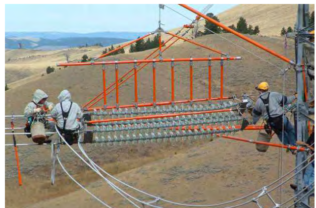
Figure 4. Live Insulator Change-out (North-western Energy UK)
