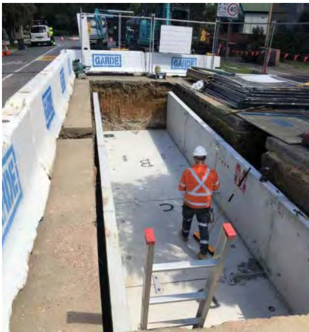
Figure 21. Powering Sydney’s Future—330kV Cable Joint Bay (Transgrid)
