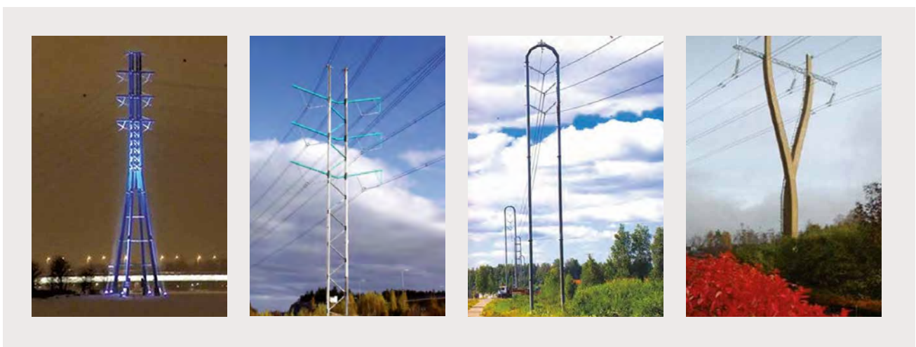
Figure 7. Examples of Aesthetic Design Transmission Line Structures (CIGRE 2017 [2], pp. 905–908)
