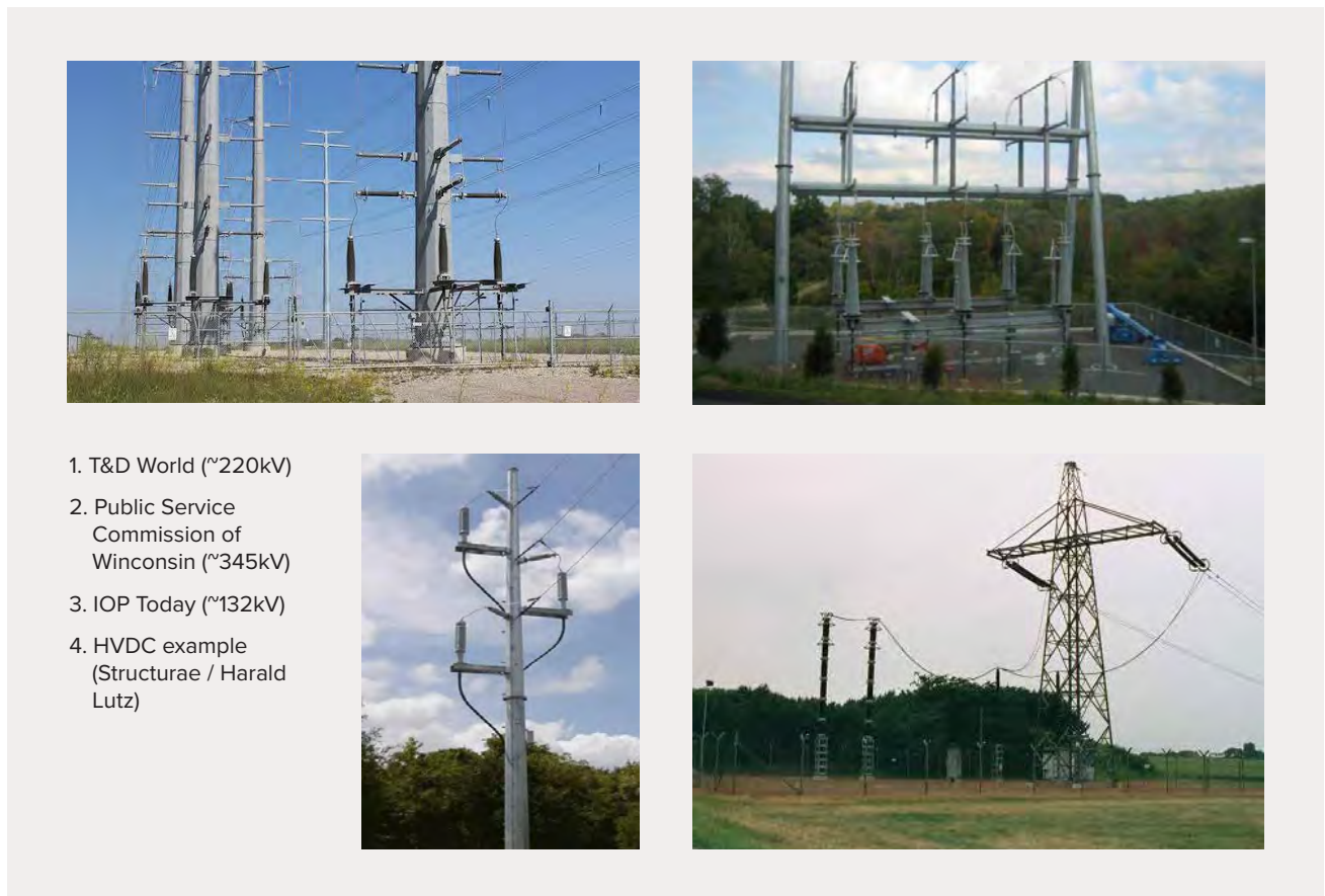
Figure 27. Examples of Overhead to Underground Transmission Line Transitions
