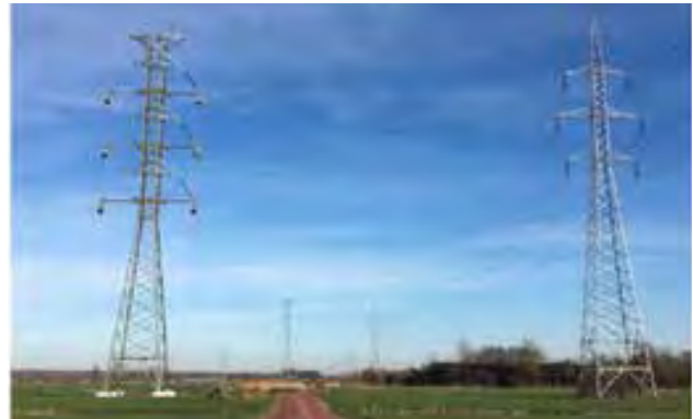
Figure 5 – Example of the tower for the compact 380 kV overhead line equipped with insulated cross-arms based on composite insulators (left) in parallel with the existing 150 kV line (right) [23]
