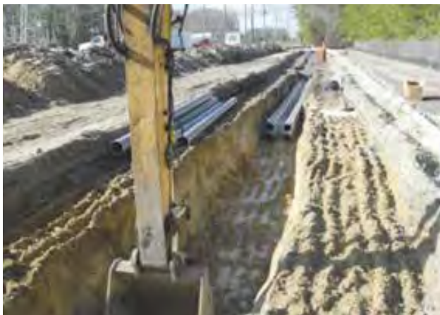
Figure 25 open cut excavation for cable system [31]
