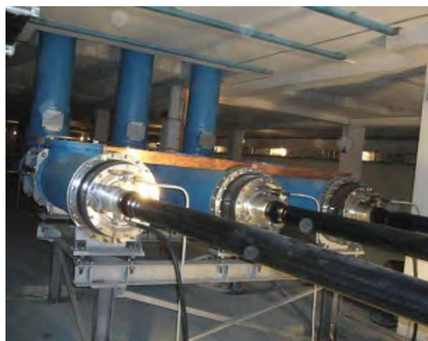
Figure 19. Typical HV Gas Insulated Switchgear (GIS) with cable terminations Installed in Horizontal Position (Nexans / Frederic Lesur)
