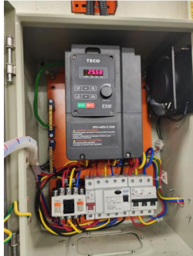
Fig 3.26. Inverter for wind speed control. Varies from 0 Hz to 50 Hz achieving wind speeds of up to 13 m/s at the outlet.
