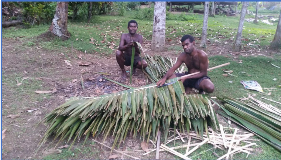
Plate 8.14: Landowners sewing sago leaves for thatching roofing.
