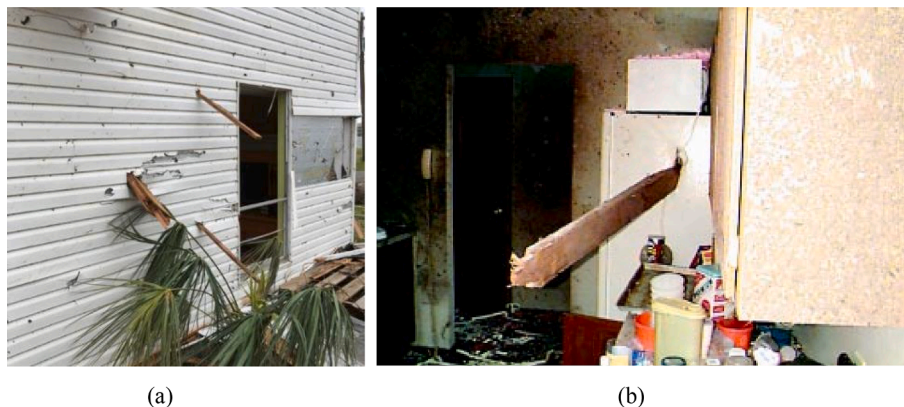
Fig. 2. Windborne debris impact: (a) Hurricane Harvey (2017) in Texas Coast [15], and (b) Tornado Alley (1999) in Oklahoma and Kansas [16].
