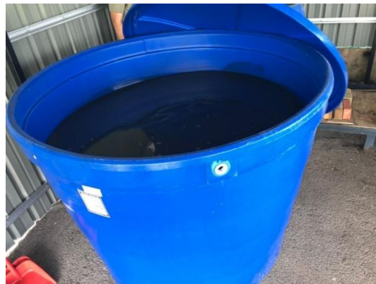
Figure 3.8: Septic sludge storage tank.
