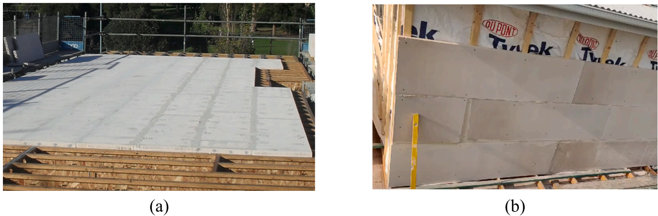
Fig. 1. 50 mm-thick reinforced AAC panel: (a) flooring panel [19] and (b) cladding panel [20].
