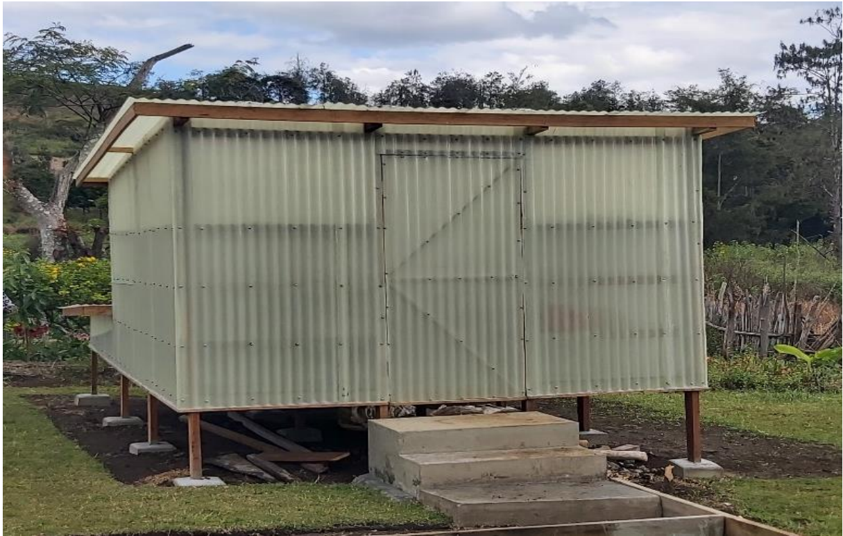
Figure 8-13 Solar dryer for bulb onions (Bena 2023)
