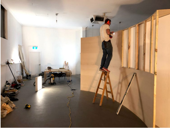
Figure 8. Installing the diorama-esque curve, Paper Mountain, 2019. Photo: Larissa Lösch.
