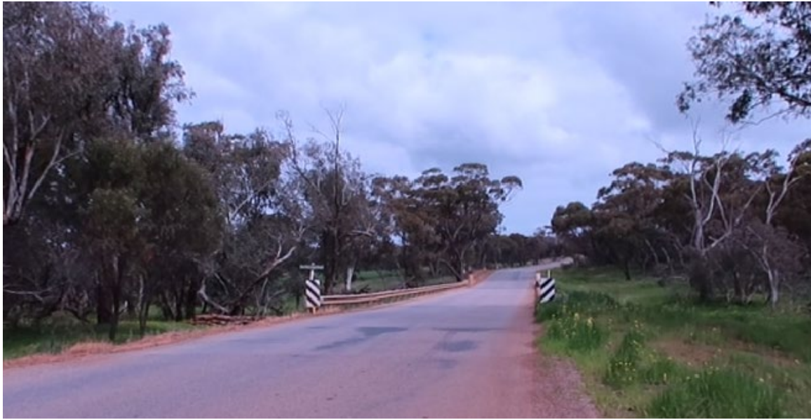
Photo 4. Rusty Bridge, Kweda Road, Brookton, 2023.
